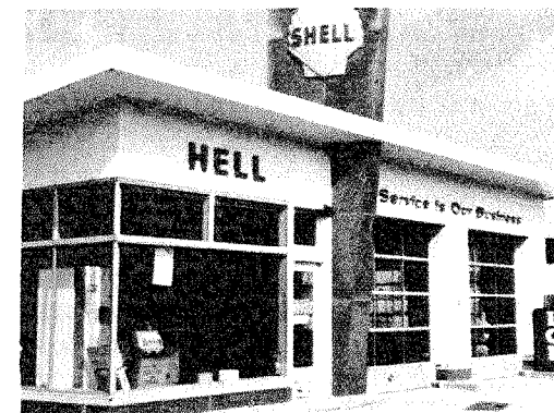
FIGURE 12—The Shell Oil Company's "S20B" station, an early example of a modified "Oblong Box."
