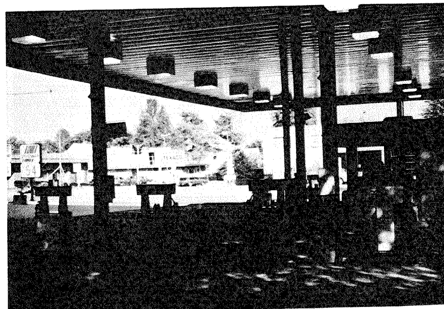
FIGURE 16— A "Canopy and Booth" station viewed from beneath the canopy.
