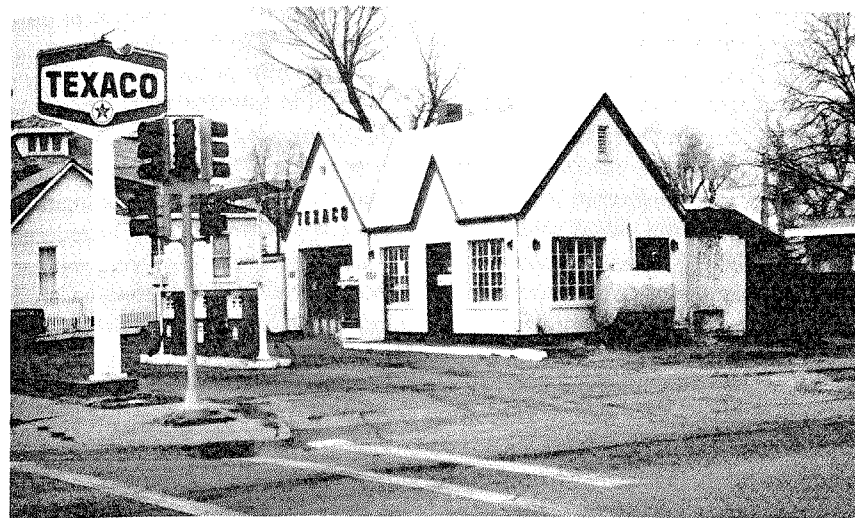
FIGURE 9 —A "House With Bay" station.
