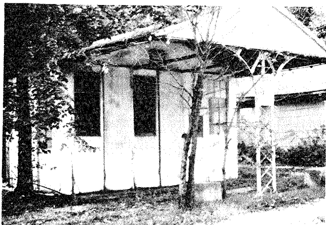
FIGURE 8 —A prefabricated "House With Canopy" station on old U.S. 66 at Wilmington, Illinois. This and similar buildings were used extensively by Standard Oil of Ohio and Standard Oil of Kentucky among other companies.
