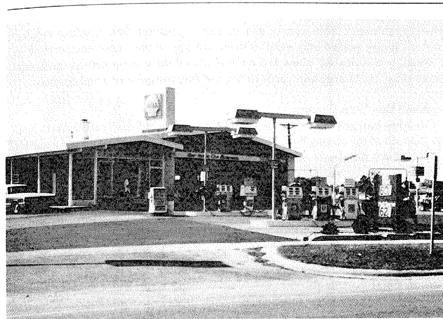
FIGURE 13— The results of "face-lifting" and "top-hatting": an "Oblong Box" modified in the "ranch style."
