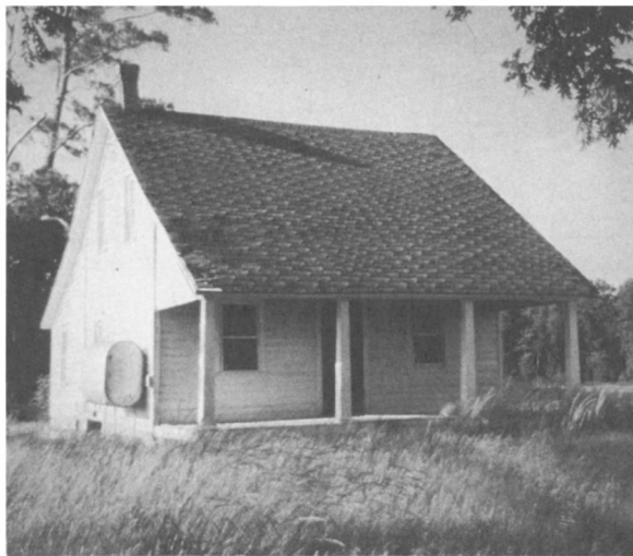
Fig. 14.2. McCabe Bungalow Exterior, Roxana Vicinity, Delaware.
